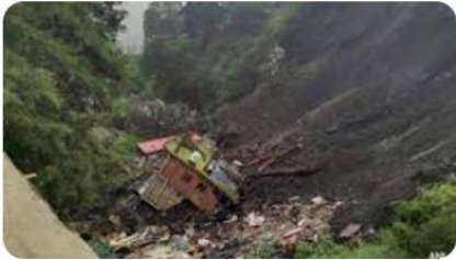
Landslide-Hit Krishna Nagar In Shimla ...
